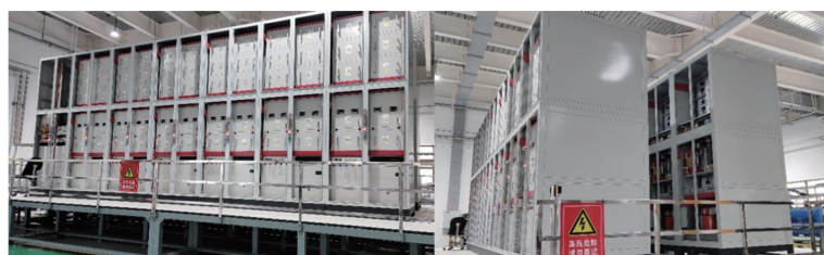
Fig. 2 (color online) The image of one set of the dipole magnet power supply system.
