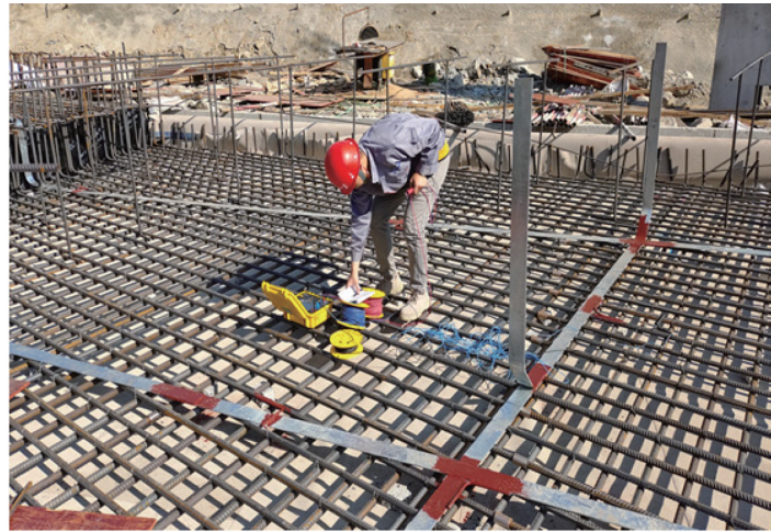
Fig. 8 (color online) Building and testing of grounding grid.
