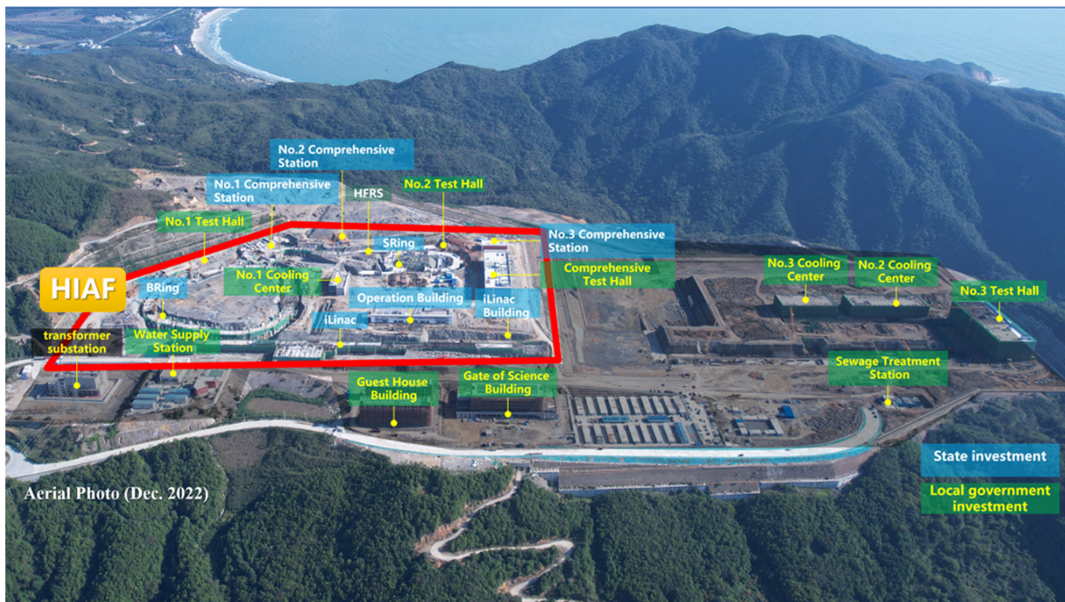
Fig. 1 (color online) The Aerial view of HIAF campus by the end of 2022 (The buildings with yellow labels are supported by local government, and those with white labels are supported by National Investment).
