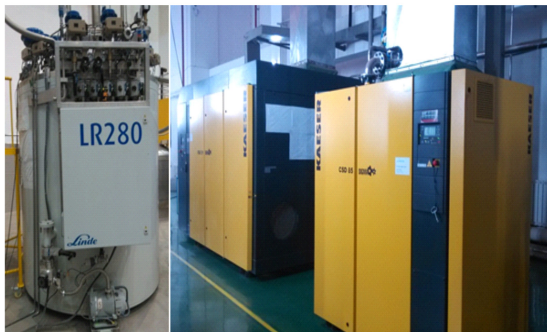
Fig. 1 (color online) Main parts of helium refrigerator system.
