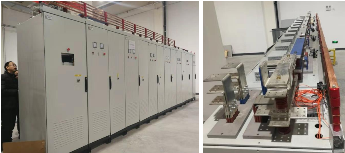
Fig. 3 Prototype of the full energy storage fast cycling pulse power supply (left) and the connections (right)
