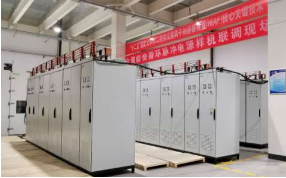
Figure 2.2 Prototype of the full-energy-storage fast-cycling pulse-power
