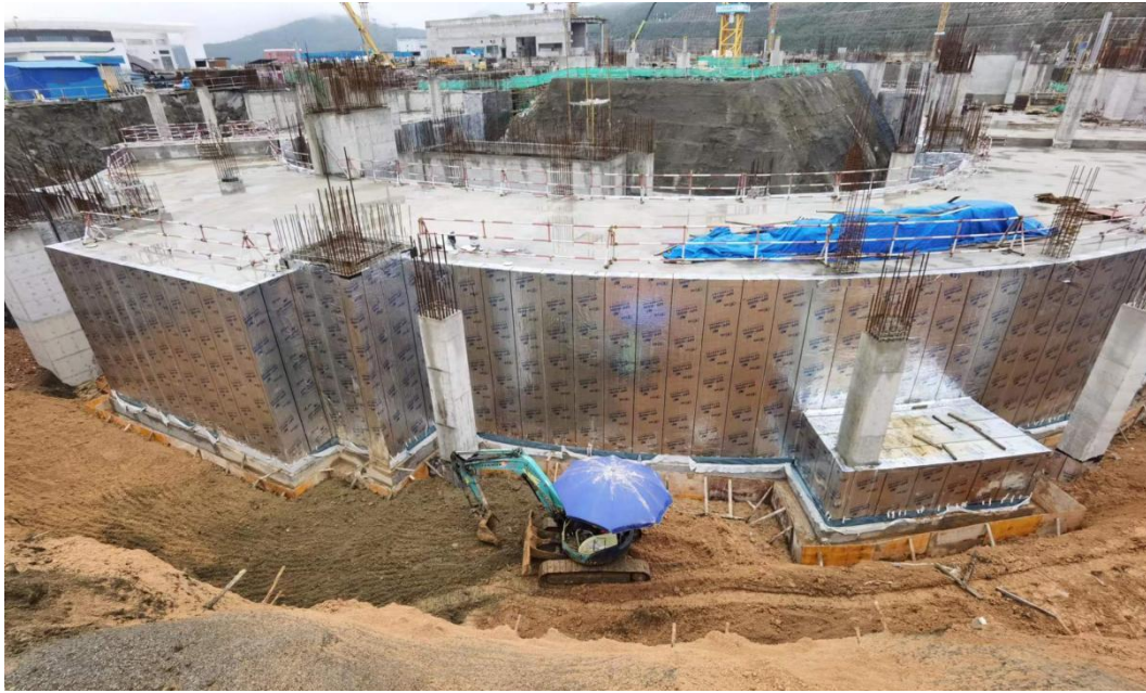
Figure 2.26 HIAF-SRing tunnel under backfilling
