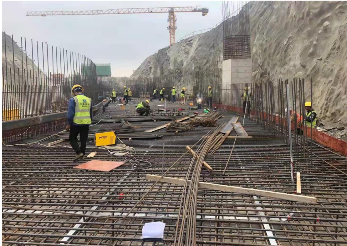
Figure 2.29 Reinforcement binding of HIAF accelerator tunnel bottom plate
