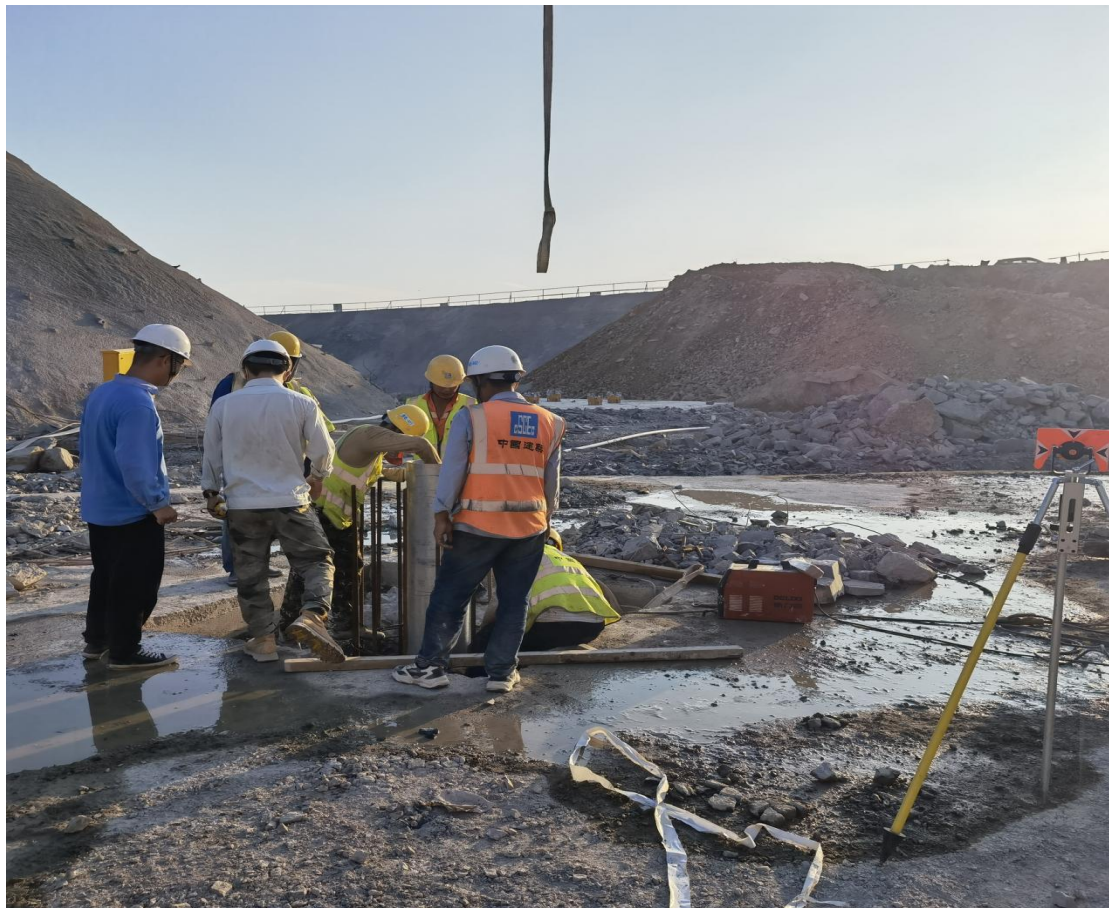
Figure 2.28 Acceptance of HIAF accelerator tunnel collimating pile
